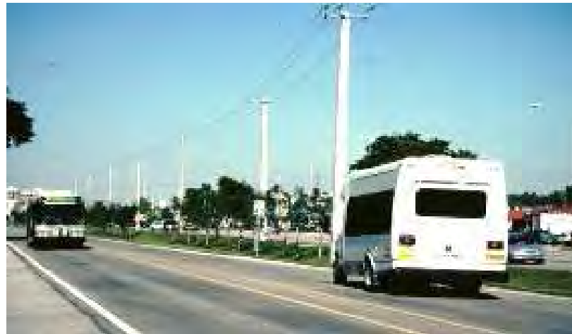
Figure 2-30 Miami's South Miami-Dade Busway, a bus-only roadway constructed in a disused rail right-of-way adjacent to an arterial.
