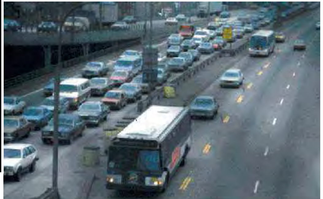
Figure 2-32 Buses and carpools bypass traffic congestion on expressways by using a contraflow HOV lane
