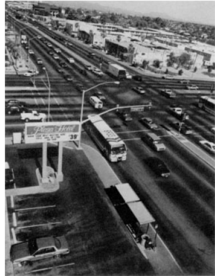
Figure 2-17 Bus stop zone design: queue jumper bus bay
