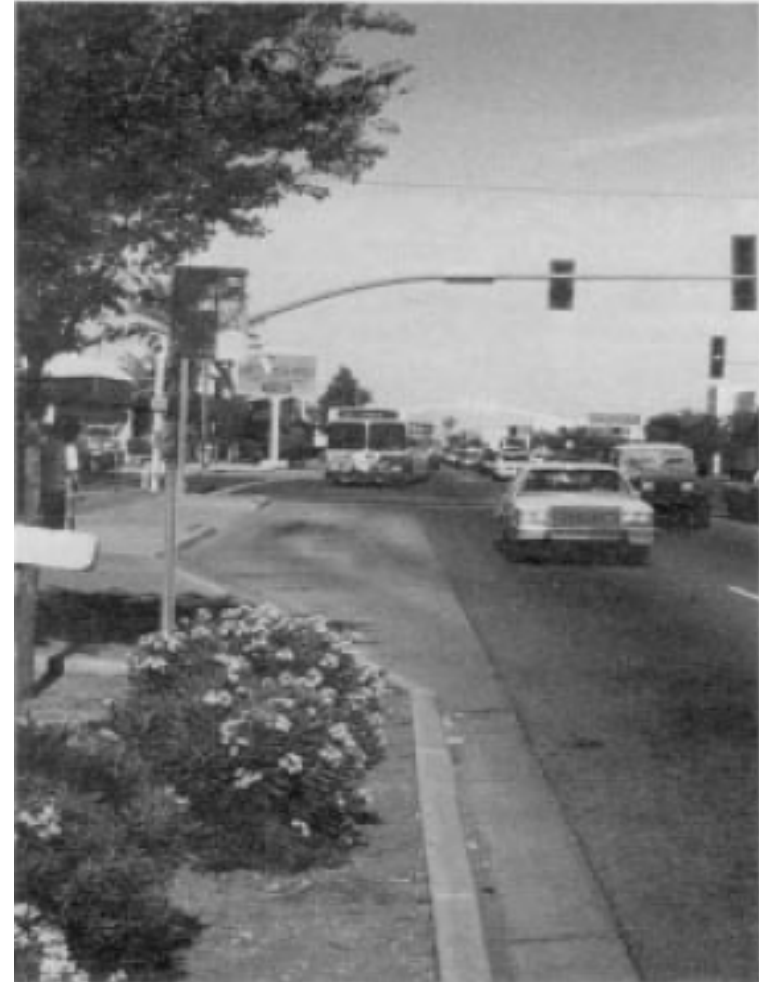
Figure 2-16 Bus stop zone design: open bus bay
