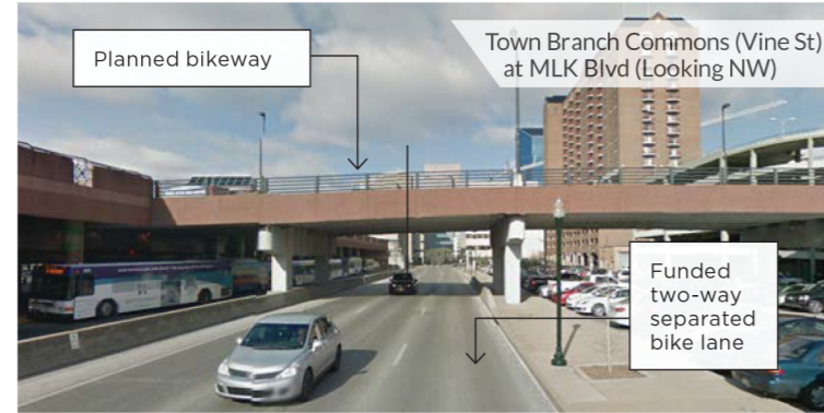
Providing a connection to from MLK to Town Branch Commons (on Vine St) requires overcoming a significant grade change from the MLK overcrossing.
