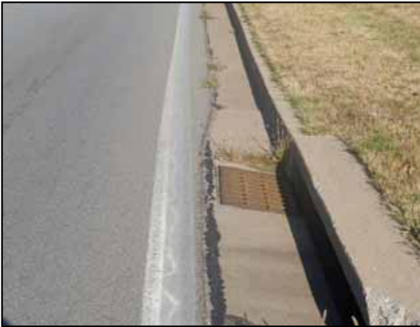
Figure 8. Damaged curb inlet and drain, and patches of grass needing trimmed.
