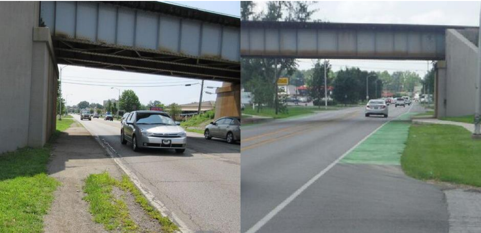
Before and after of a sidewalk and bike lane installation project.
