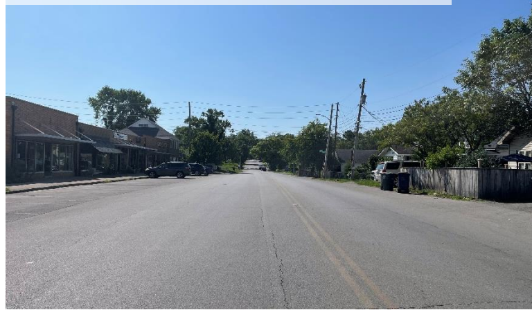
Liberty Road near Winchester Road (looking southeast)
