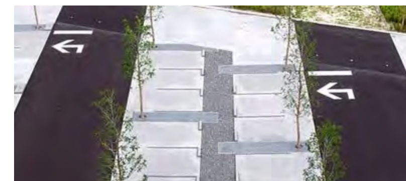
Green infrastructure integrated into parking lot
